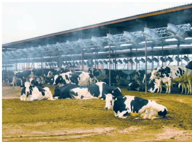
In side-by-side tests against other leading arid climate dairy cooling systems, FlipFan provides equal or greater cow cooling, using less electricity and less water.
